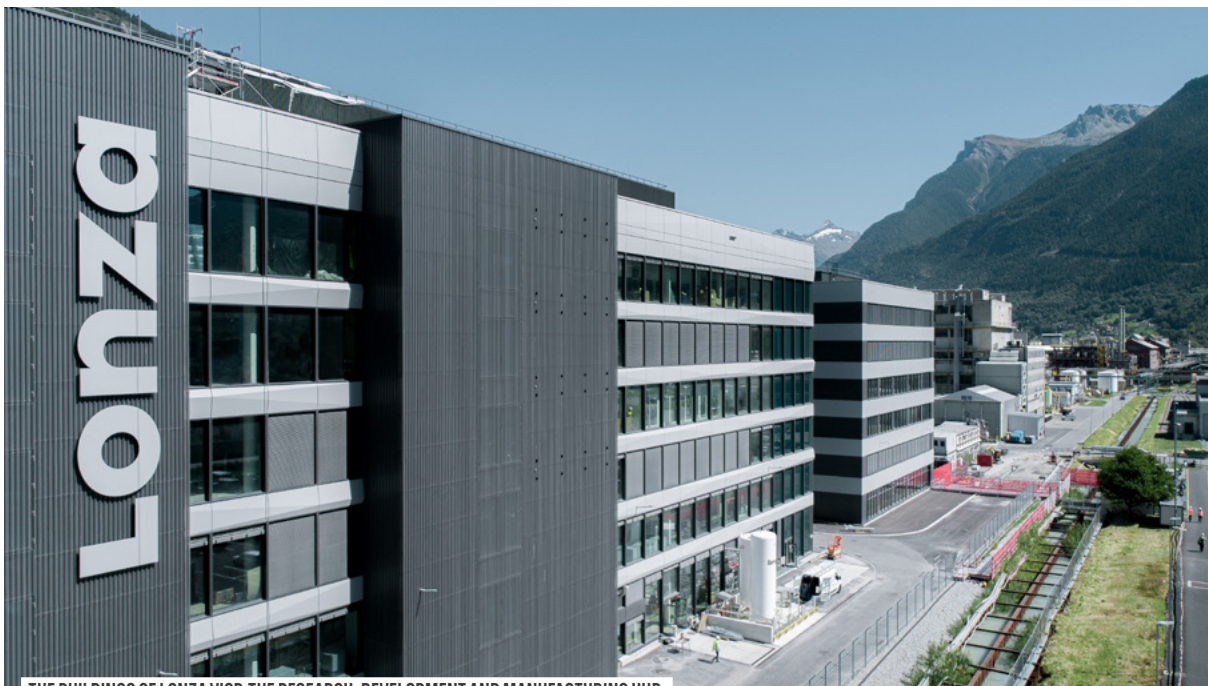
THE BUILDINGS OF LONZA VISP, THE RESEARCH, DEVELOPMENT AND MANUFACTURING HUB.
