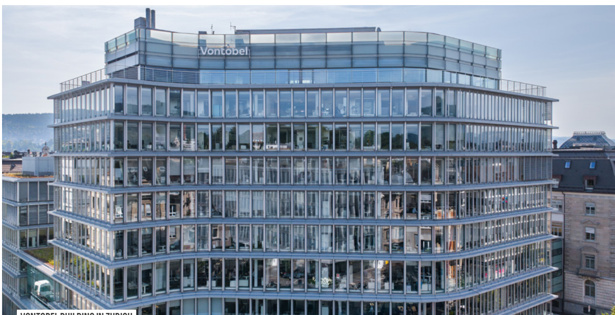
VONTOBEL BUILDING IN ZURICH
